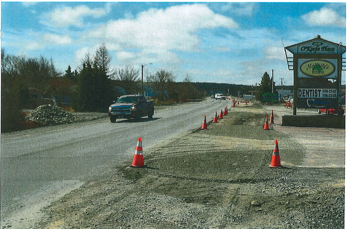
Fig 14. Sidewalk construction in Carbonear on May 2 2023.
